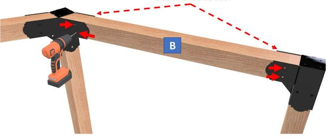
4. Drive one ½ x 1-1/4" Lag Screw through each 5/16" hole into the pilot holes you drilled in step 3, using a 7/16" Socket and Rachet driver. Tighten down each screw.
