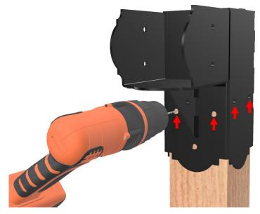
4. Drive one ¼ x 1-1/4" Lag Screw through each 5/16" hole into the pilot holes you drilled in step 4, using a 7/16" Socket and Rachet driver. Tighten down each screw.
