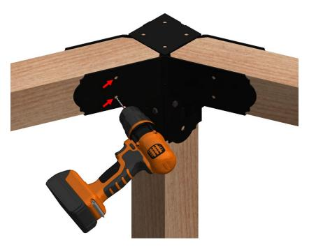
4. Drive one ¼ x 1-1/4" Lag Screw through each 5/16" hole into the pilot holes you drilled in step 8, using a 7/16" Socket and Rachet driver. Tighten down each screw. Repeat for opposite side of the U-channel and the opposite end of the header.
